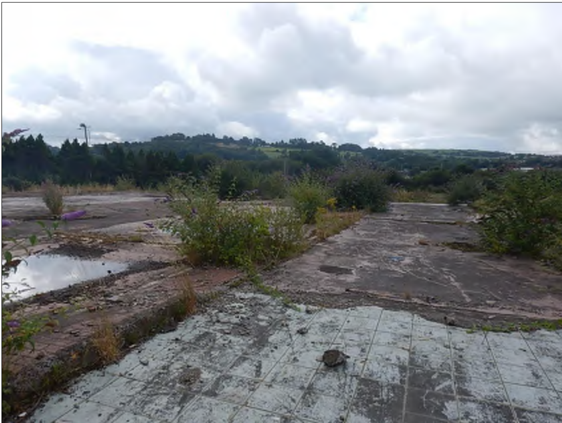
Plate 6: Floor levels of former buildings in central area of proposed development site, looking south
